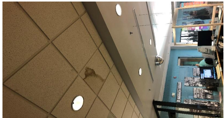
Leaks over costly technology
